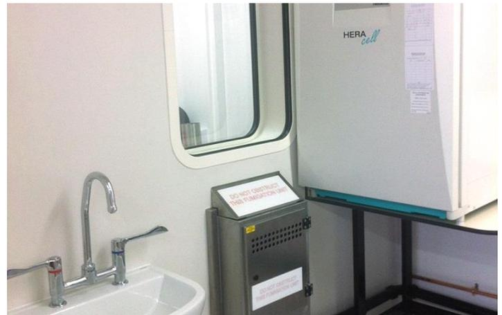
To provide an easy and safe way of fumigating the main laboratory, Enbloc installed a fumigation chamber, that was wall mounted between the lobby and main room. This allows the users to place the fumigant in the chamber from the laboratory and energise the fumigation chamber from the lobby meaning no users need to enter the laboratory during the entire fumigation cycle. A test port installed to the suite door allows the users to check fumigant levels before re-entering the laboratory.
