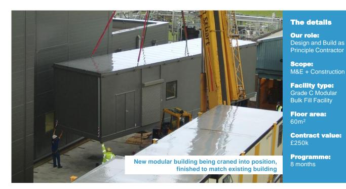
Through negotiation on Enbloc's Partnership scheme, the contract for Avecia's new modular bulk fill facility was a welcome challenge for Enbloc. Avecia required an extension to their ABC2000 plant to match visually both internally and externally. The brief included a preference for the extension to be modular and, therefore, built and fitted-out off site; Enbloc designed a painted steel module to match the existing grey facades.
