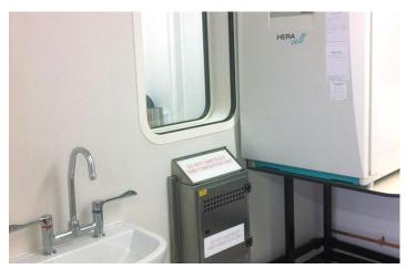
To provide an easy and safe way of fumigating the main laboratory, Enbloc installed a fumigation chamber, that was wall mounted between the lobby and main room. This allows the users to place the fumigant in the chamber from the laboratory and energise the fumigation chamber from the lobby meaning no users need to enter the laboratory during the entire fumigation cycle. A test port installed to the suite door allows the users to check fumigant levels before re-entering the laboratory.
