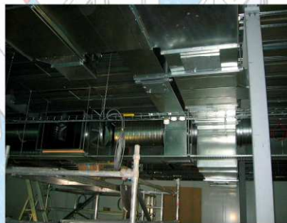
Installation of ductwork in ceiling void under new mezzanine.
