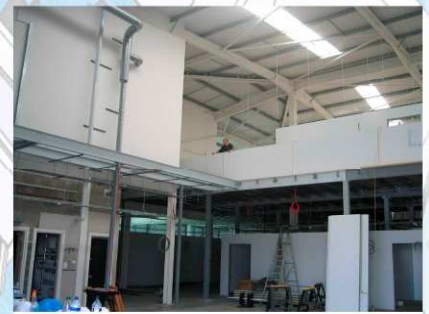
Constructing cleanroom panels over two floors.
