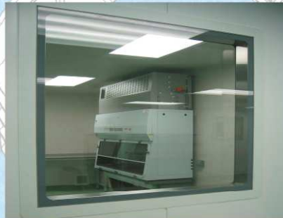
Flush fit cleanroom vision panel allowing viewing of grade B extract cleanroom.
