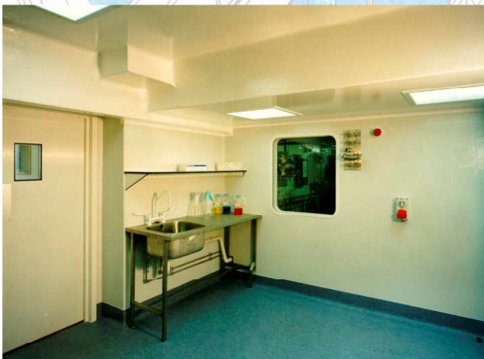
Full GRP Interior finish of containment suite.
