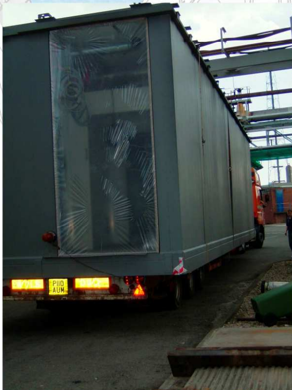
Portable cleanroom being trucked to site with panel walls, electrics, pipe work and HVAC already installed
